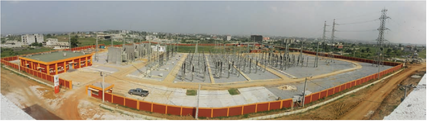
225/16.5kV Djibi substation, Ivory Coast
