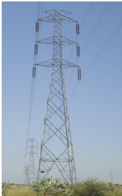
220kV Gadaref-Gallabat transmission line, Sudan
