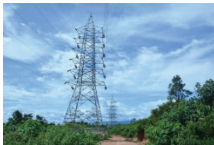
115kV multi-circuit line, Laos
