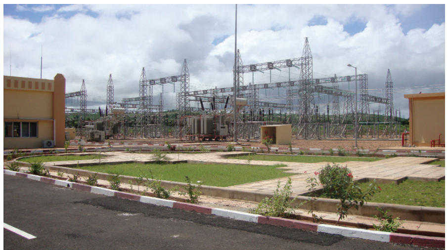
225/30/15kV Sikasso substation, Mali
