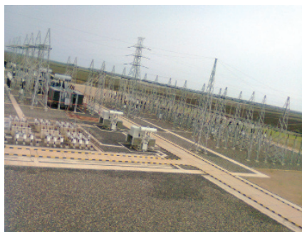
220/110/33kV Singa substation, Sudan
