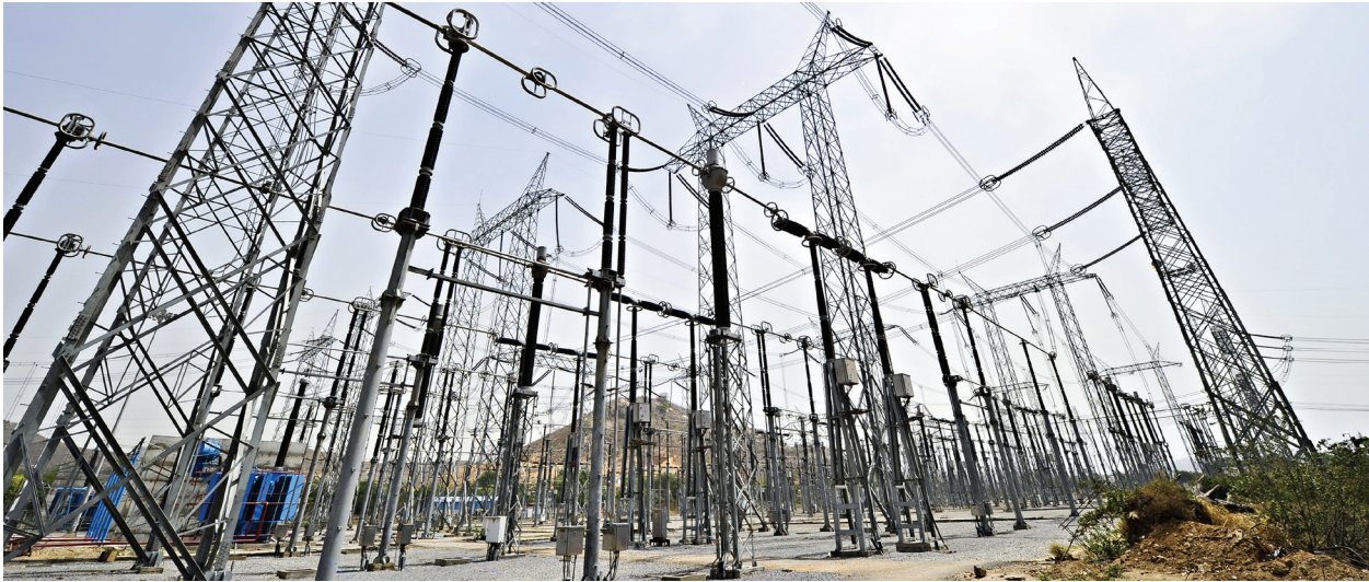
Technology wise India is migrating to higher transmission voltages, working on bulk transmission and has a fully synchronised national grid.
