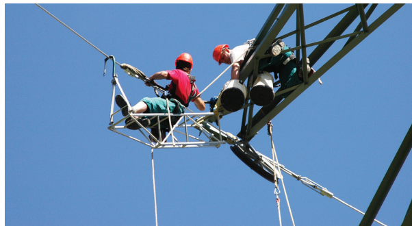
In India, T&D losses account for as high as 23 per cent of the total electricity generated
