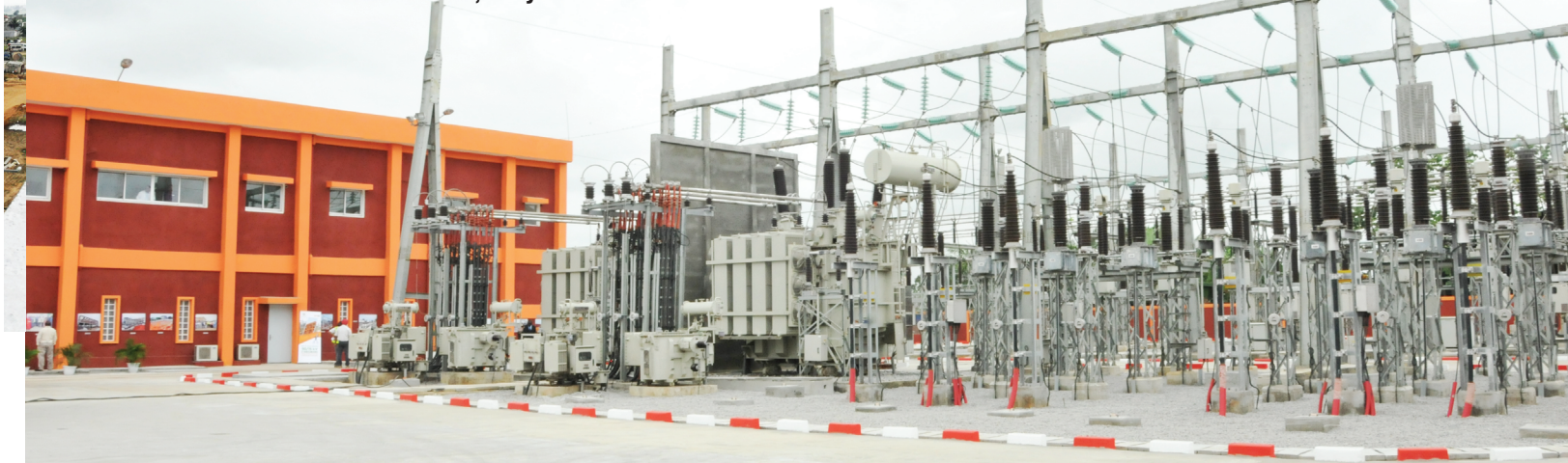
90/15 KV Anoumabo Substation, Ivory Coast
