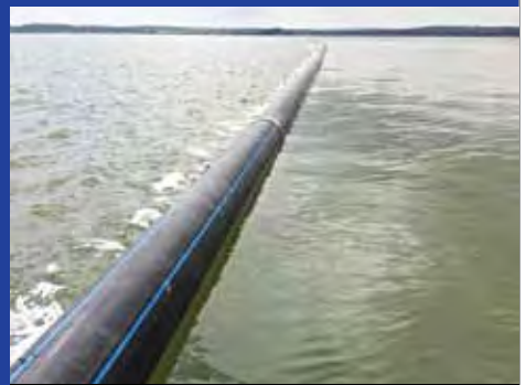
Water Supply System, Tanzania
