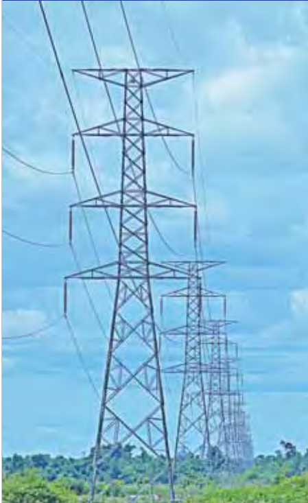
230 KV Transmission line, LAOS
