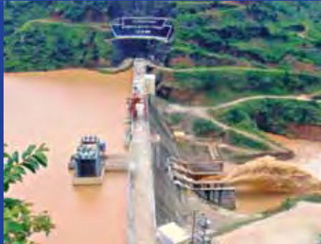
Nyabarongo, Hydropower, Rwanda
